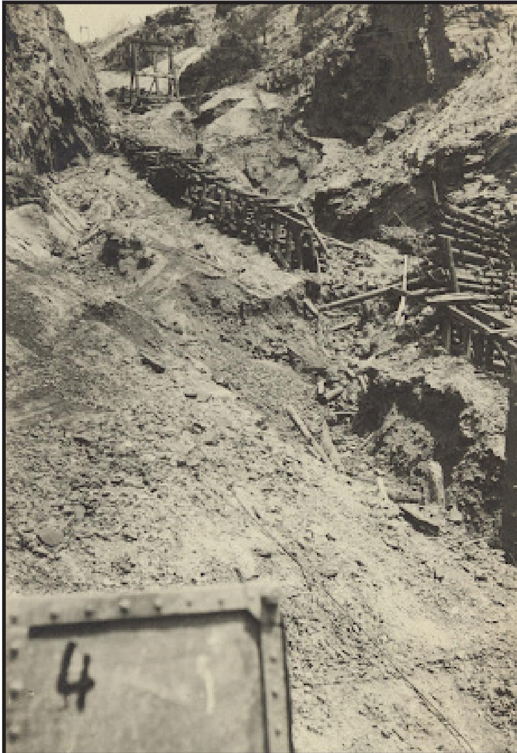
(1916) Damage to cribbing and tramway at Belden from a mudslide.
