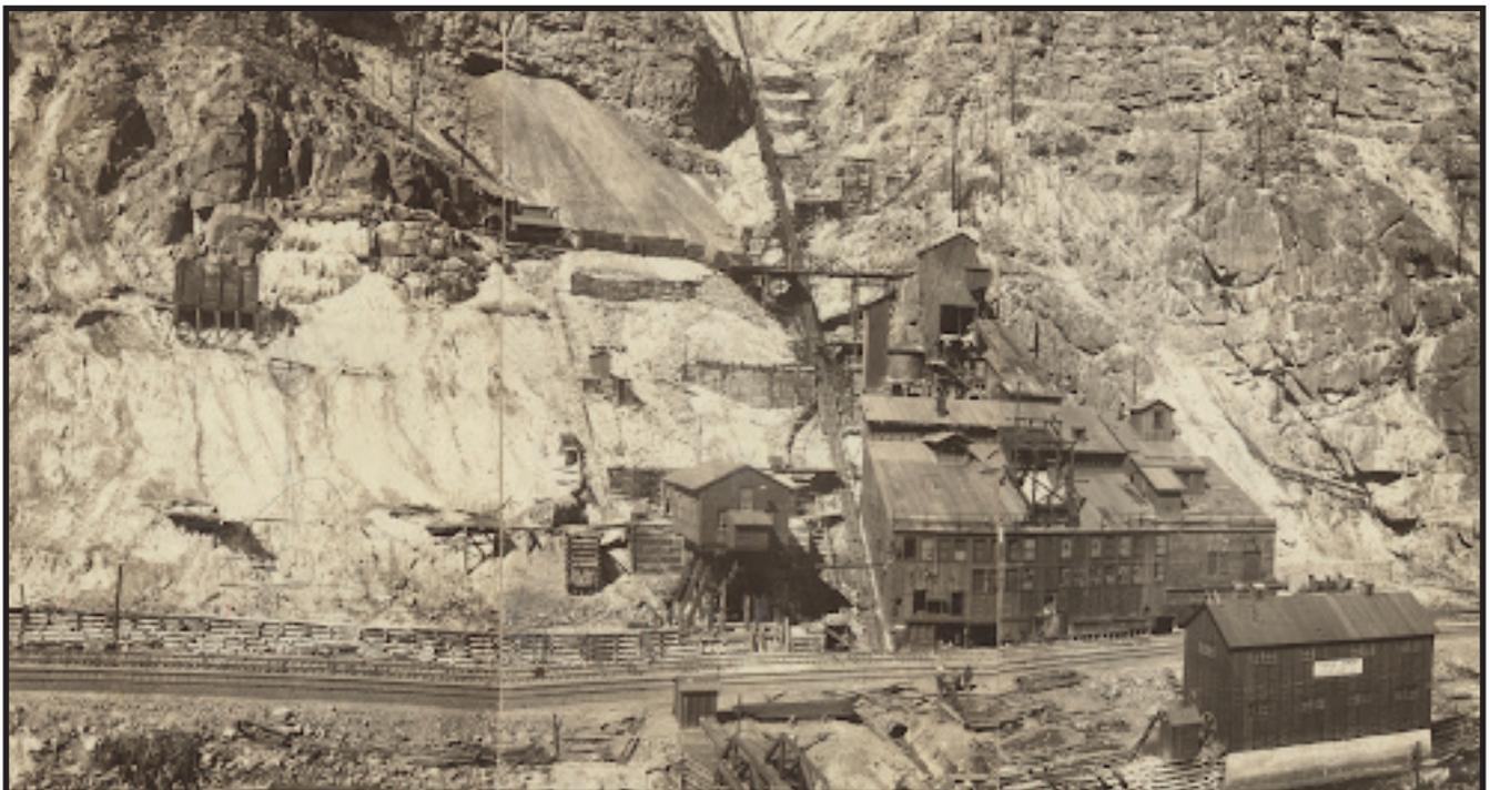
(1927) Belden as seen in 1927 under the control of Empire Zinc. The new Copper Tipple loading dock is visible in the lower center, the surface tram is to the right, and the processing buildings are to the right of that. Across the railroad tracks is the hardware building with a sign on it reading: "Eagle Mines of the Empire Zinc Co." Men are visible working on the tracks in front of the processing buildings. *Gilman Photograph Collection, Colorado School of Mines Repository.*
