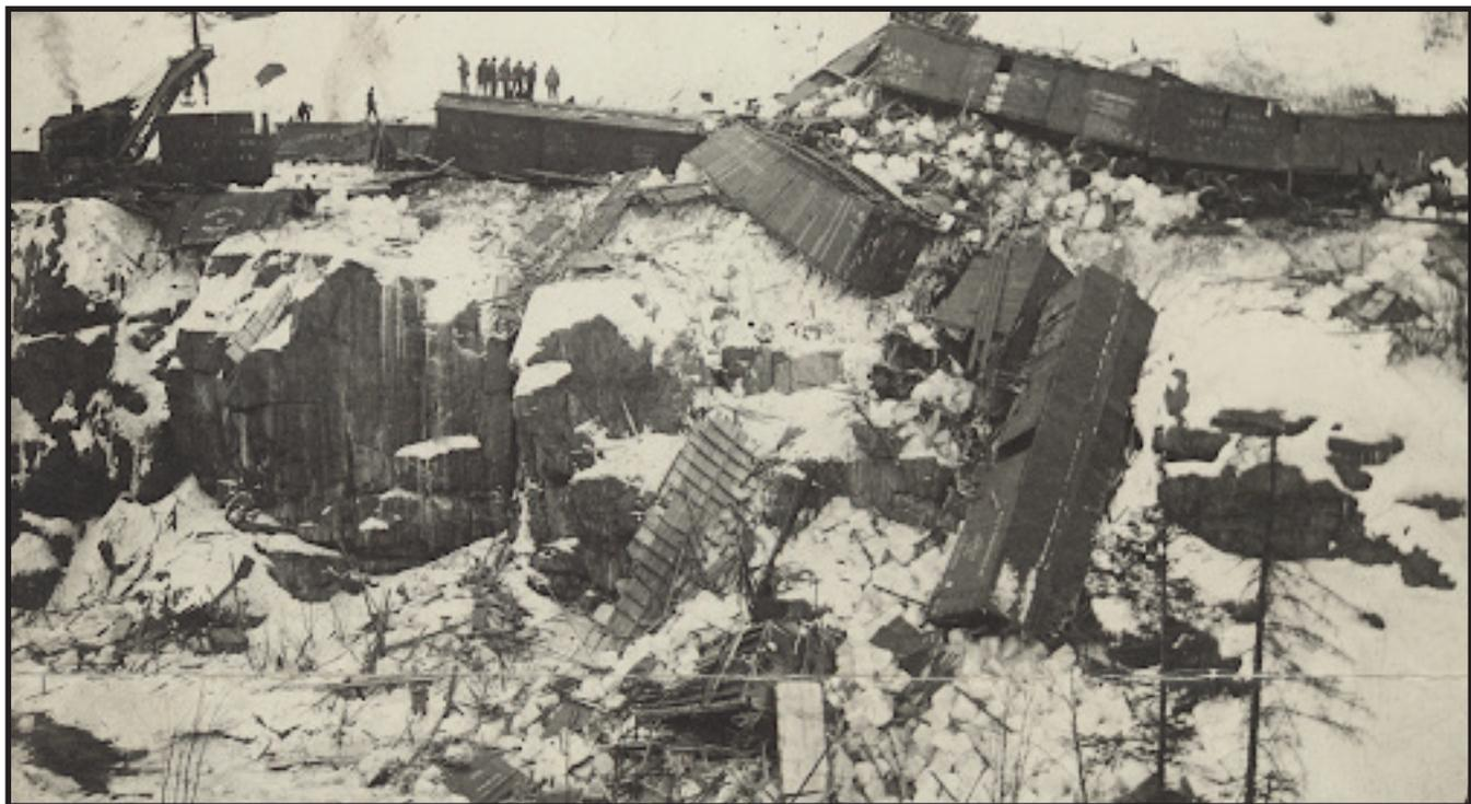
(1918) A severe train wreck and derailment just northwest of Belden by Rock Creek, likely caused by winter conditions. Men are visible standing on their overturned cars. The box cars are full of ice which was likely harvested at Pando, the area that would later become Camp Hale. *Gilman Photograph Collection, Colorado School of Mines Repository.*
