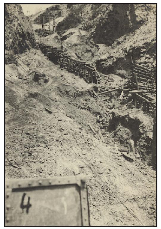
(1916) Damage to cribbing and tramway at Belden from a mudslide. *repository.mines.edu*
