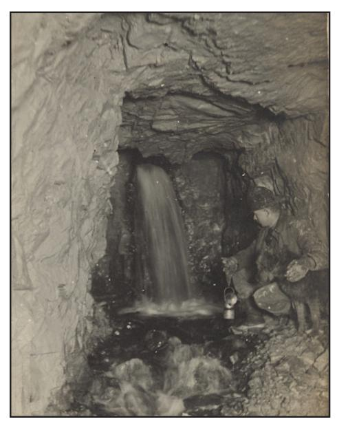
(1916) Miner inside the Newhouse Tunnel holding a lamp with his dog. Flooding was common within the mines of Battle Mountain, especially as Empire Zinc dug below the water table. *Gilman Photograph Collection, Colorado School of Mines Repository.*
