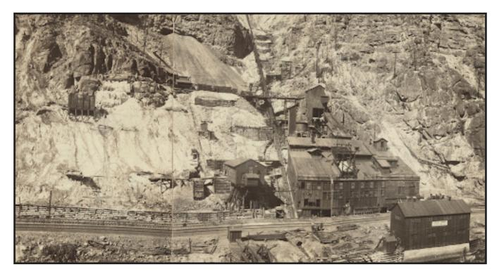
(1927) Belden as seen in 1927 under the control of Empire Zinc. The new Copper Tipple loading dock is visible in the lower center, the surface tram is to the right, and the processing buildings are to the right of that. Across the railroad tracks is the hardware building with a sign on it reading: "Eagle Mines of the Empire Zinc Co." Men are visible working on the tracks in front of the processing buildings. *Gilman Photograph Collection, Colorado School of Mines Repository.*
